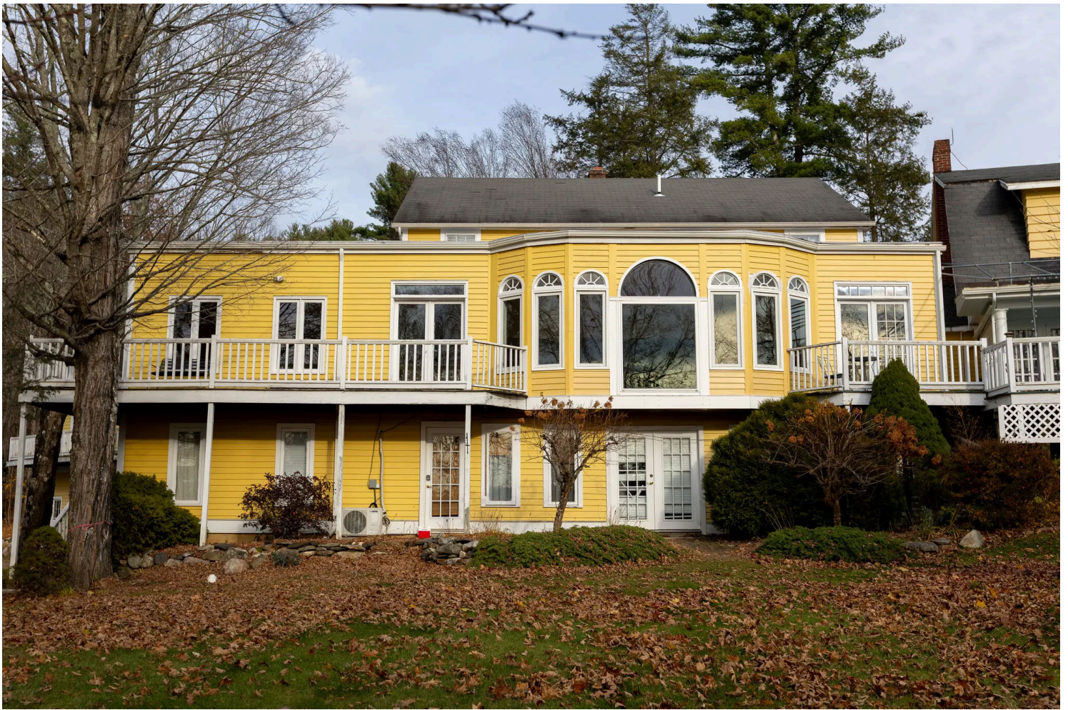
The Thornewood Inn in Great Barrington, Mass., is a former bed-and-breakfast that catered to vacationers and has been converted into worker housing. Patrick Dodson for The New York Times
